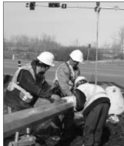
Workers re-install traffic lights on Highway 15 south of the Scotford Upgrader. Installation of the lights will be completed in advance of the Shell Scotford Upgrader spring maintenance turnaround.
